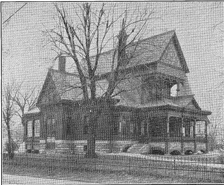
GENERAL OFFICES BUILDING AT INDEPENDENCE
