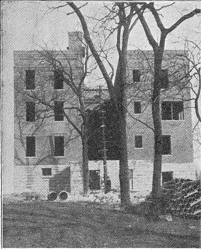
REAR VIEW OF SANITARIUM AS SHOWN IN JANUARY.
