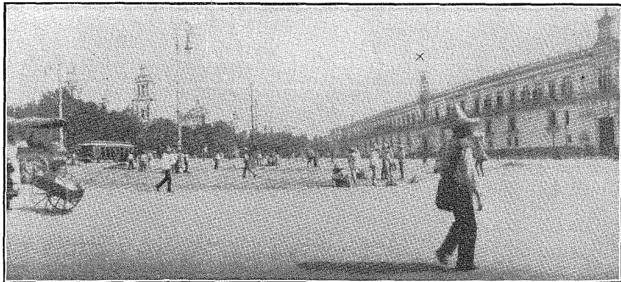
Mexican "National Palace," containing Government Buildings and Army Quarters, Mexico City.
